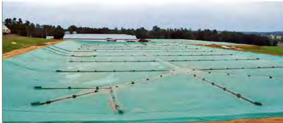
Photo of a covered anaerobic lagoon
